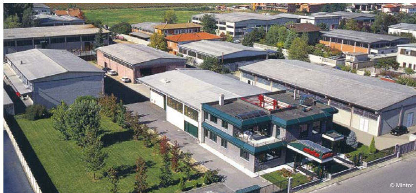
A bird's eye view of the Mintor's factory. Veduta aerea dello stabilimento Mintor.
